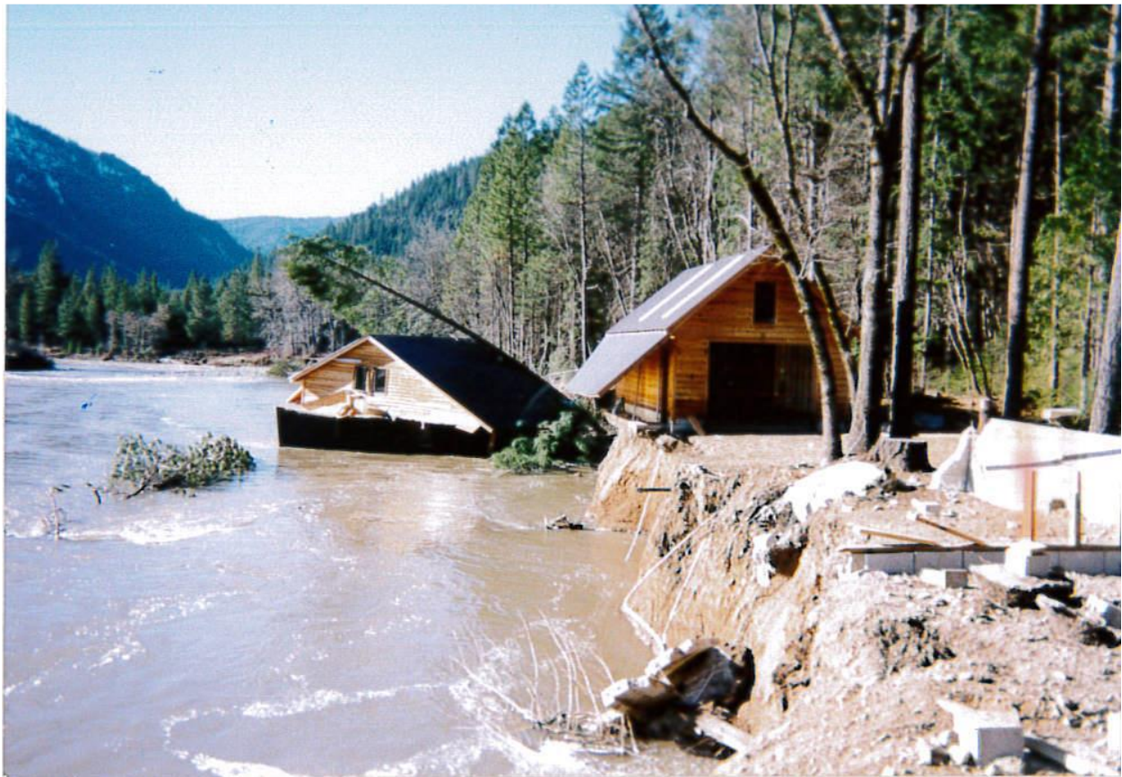
Figure 4-129 Erosion from Floodwaters Cause Home to fall into Indian Creek
