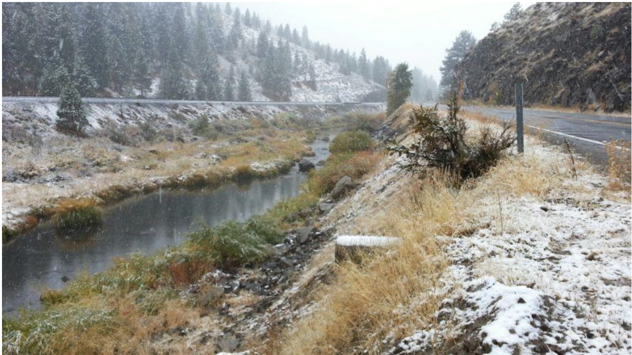
Figure 4-150 Rocky Point Road – Shoulder Erosion from Localized Flooding
