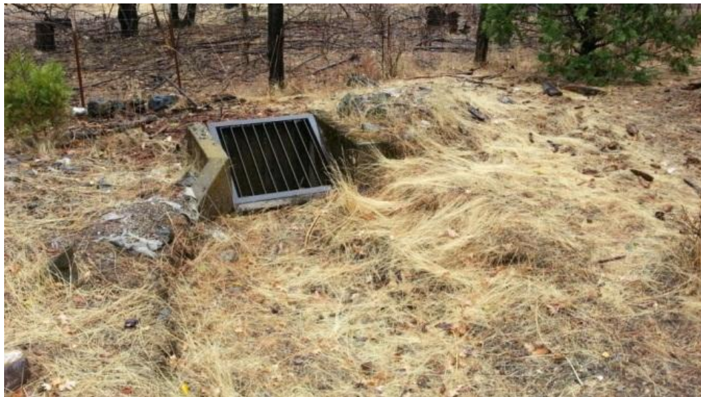
Figure 4-165 American Valley Localized Flooding – Small drain for Mill Creek can be Bypassed During Larger Storms Causing Water to Flow Down Adjacent Gravel Road.
