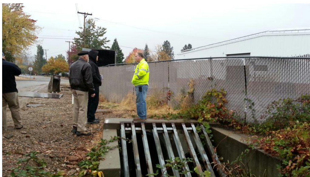
Figure 4-157 American Valley Localized Flooding – Storm Grate behind Les Schwab Becomes Clogged with Debris Causing Flooding
