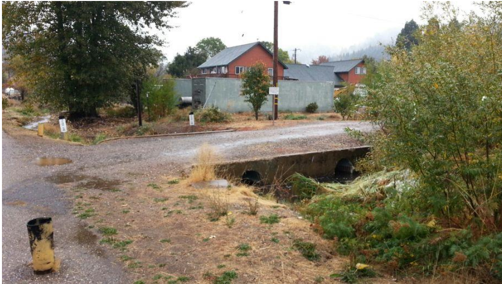
Figure 4-162 American Valley Localized Flooding – Water Overtops Drainage at Culverts Where Forced to take 90-degree Right Turn.
