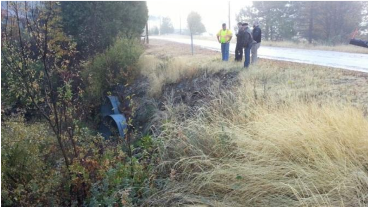
Figure 4-152 Indian Valley Localized Flooding – North Valley Road crossing Williams Creek where Culverts often Clog with Debris
