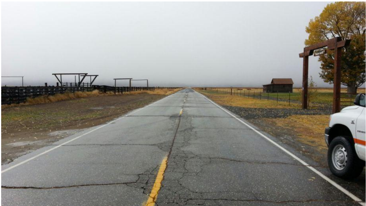
Figure 4-151 Harriet Lane – Pavement Deterioration from Localized Flooding
