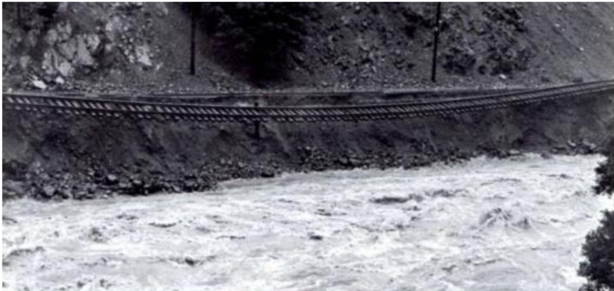
Figure 4-126 1986 Railroad Bed Flood Damages
