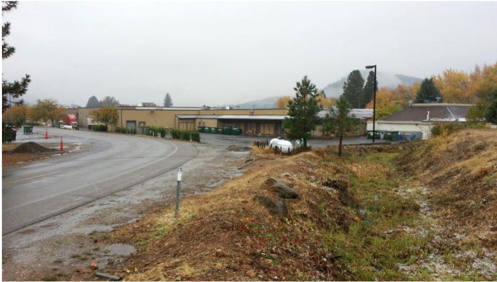
Figure 4-158 American Valley Localized Flooding – Strip Mall Containing Paradise Grill and other Businesses. Water can Overtop Earthen Ditch on Right, or Flow Down Street on Left when Storm Drain Floods behind Les Schwab
