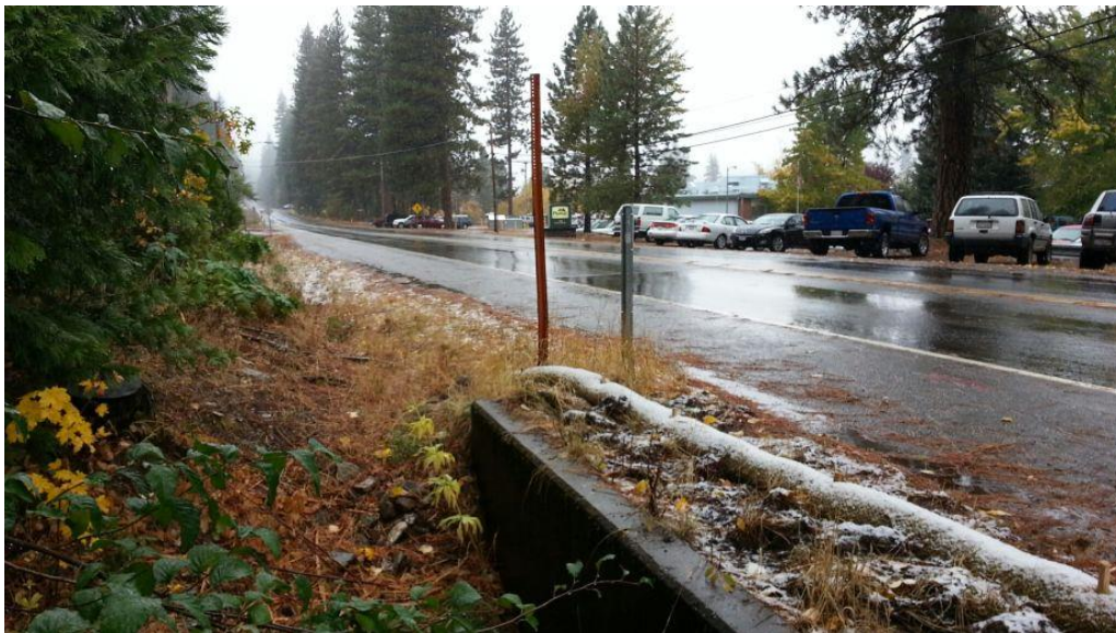
Figure 4-163 American Valley Localized Flooding – View of Plumas District Hospital from Storm Grate along Gansner Creek. Apparent that Hospital is Down Slope from Culvert and Subject to Flooding from Overtopping Water.
