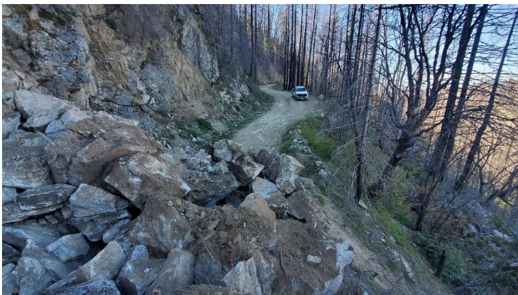
Figure H-9 Rockslide Debris Slides Blocking Roadway to Dam – Alternate view
