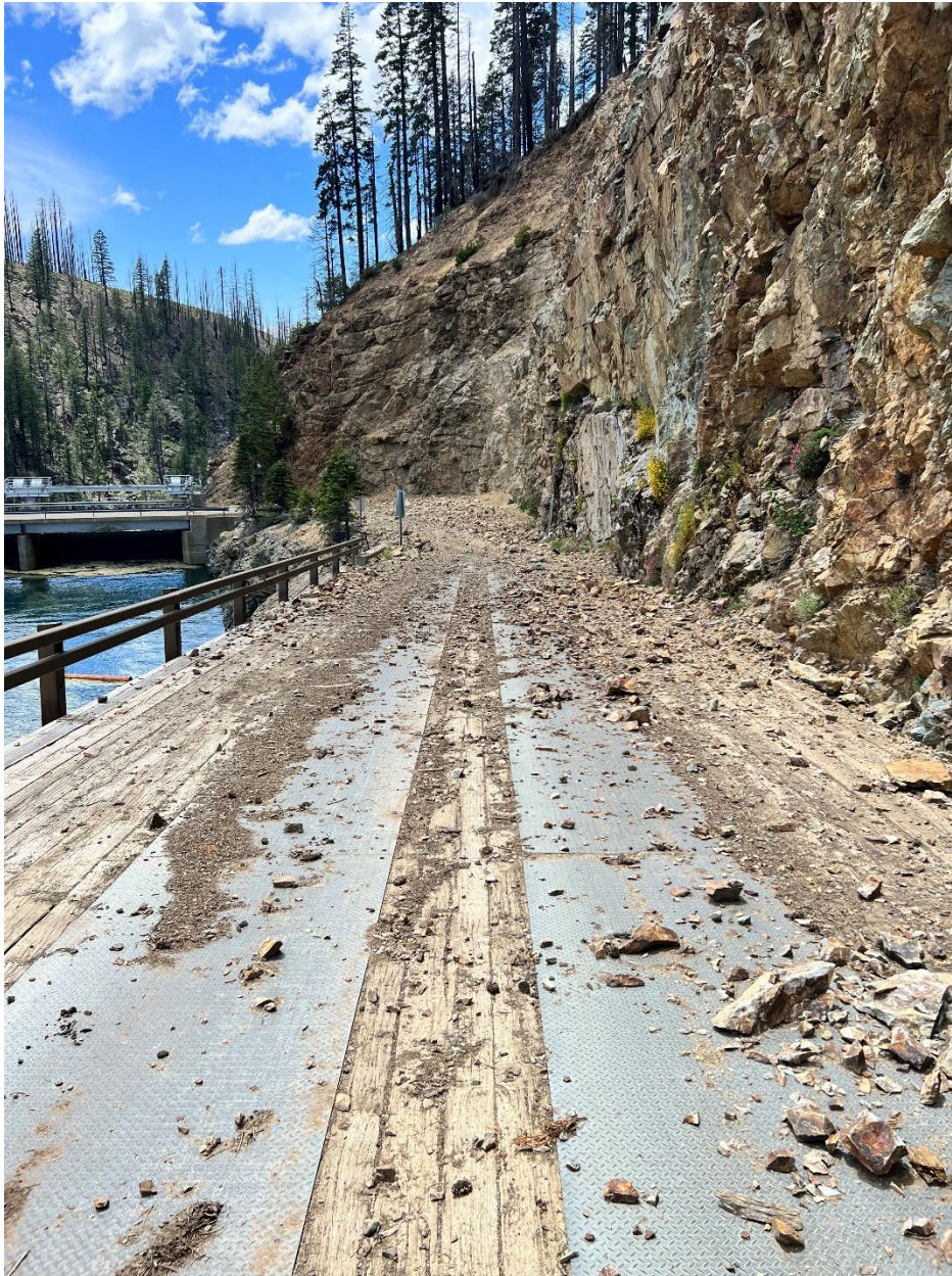
Figure H-11 Debris Slides Post North Complex Fire Above Little Grass Valley Dam – Alternate view
