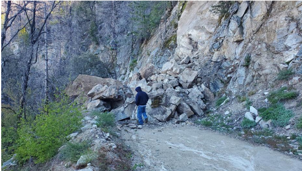
Figure H-9 Rockslide Debris Slides Blocking Roadway to Dam – Alternate view
