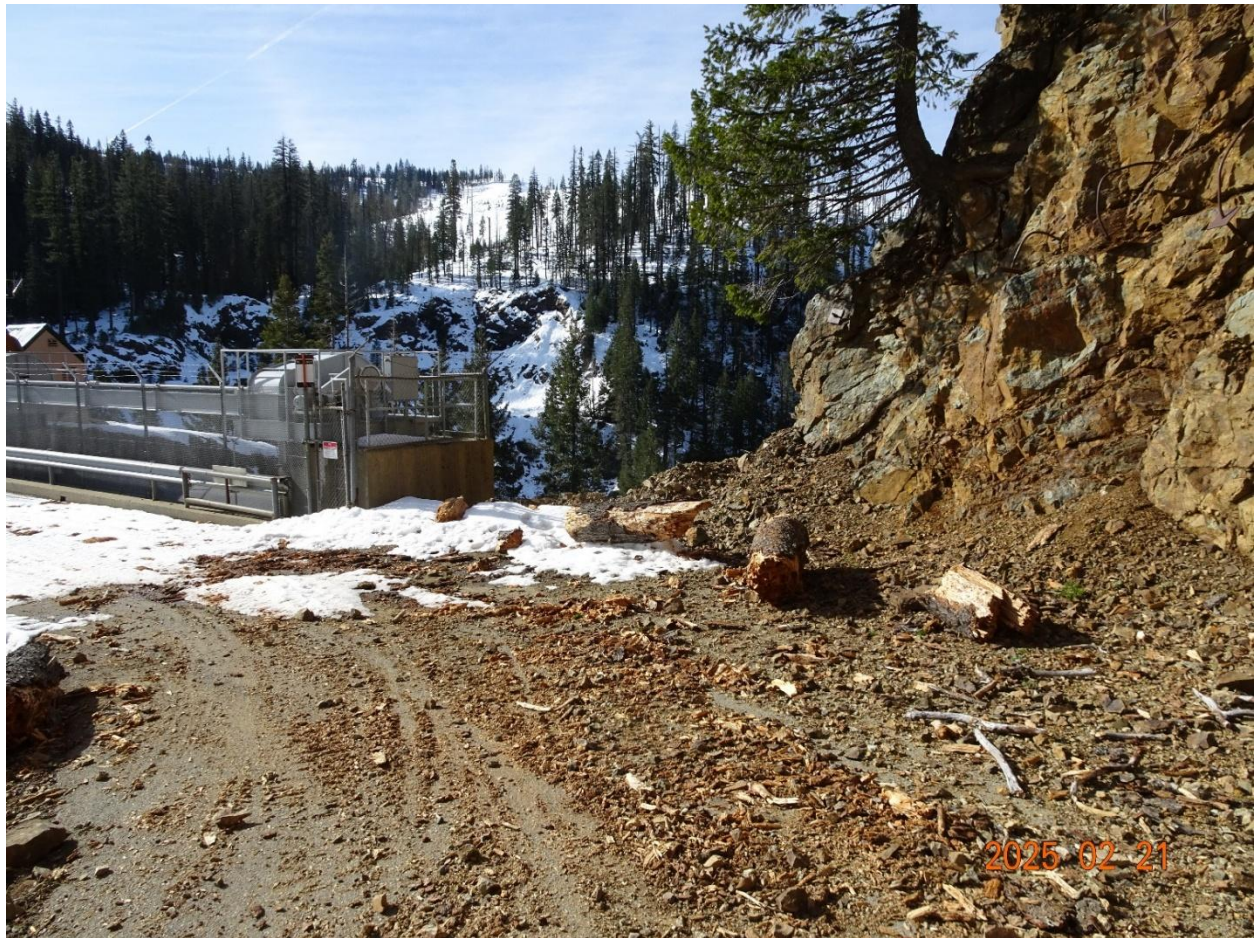
Figure H-10 Debris Slides Post North Complex Fire Above Little Grass Valley Dam
