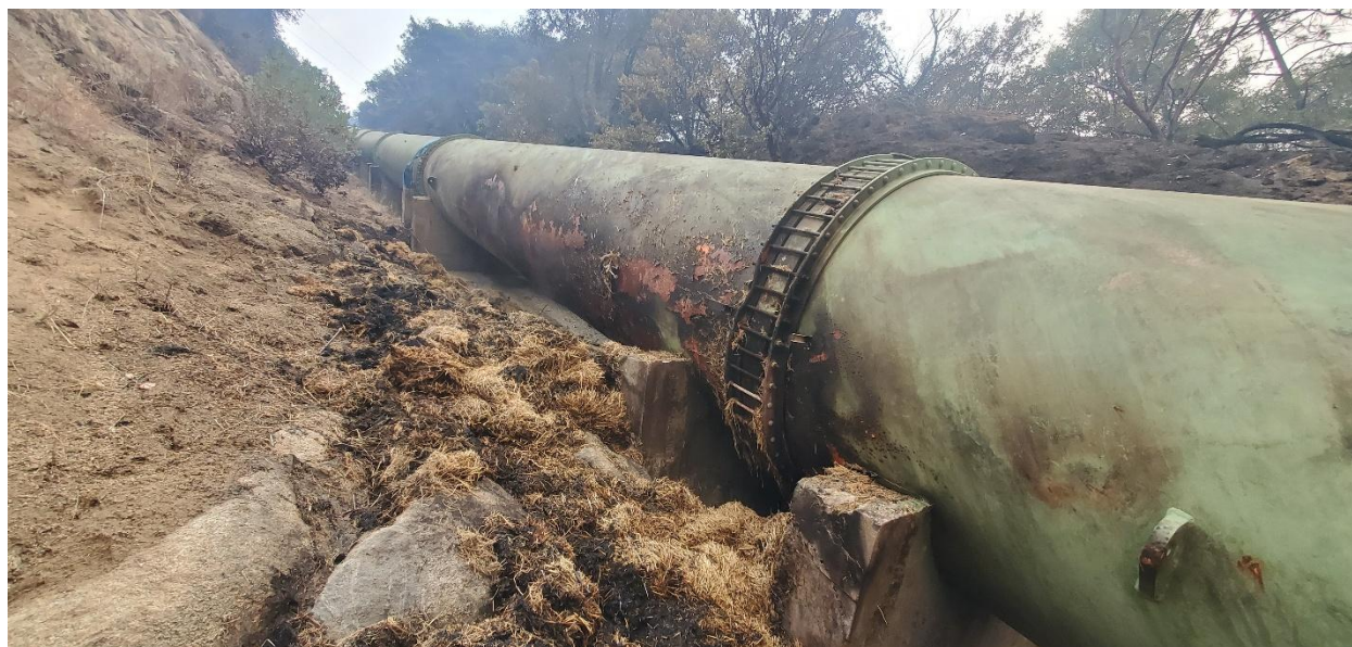
Figure H-14 Burns on Piping from North Complex Fire
