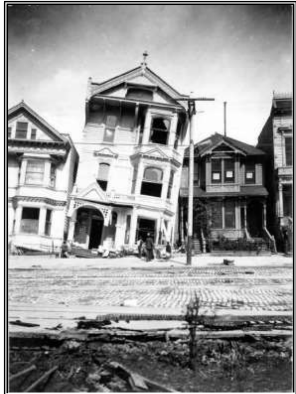
Image 5 – Results of Liquefaction in 1906
