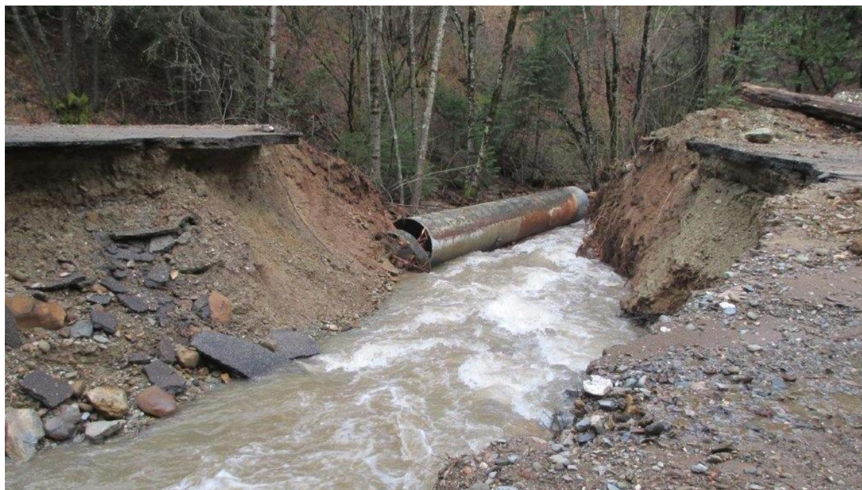
Figure 4-107 Plumas County – Thompson Creek Washout
