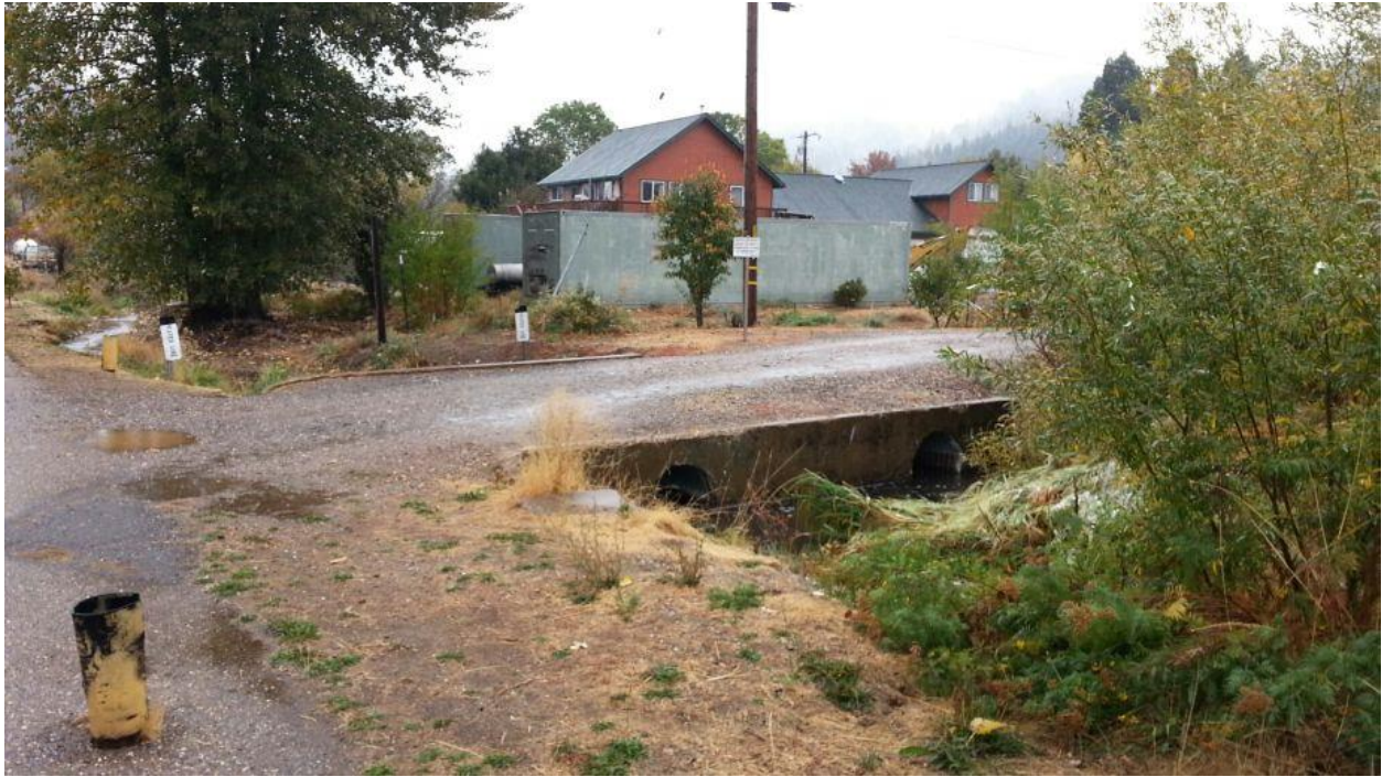
Figure 4-128 American Valley Localized Flooding – Water Overtops Drainage at Culverts Where Forced to take 90-degree Right Turn.
