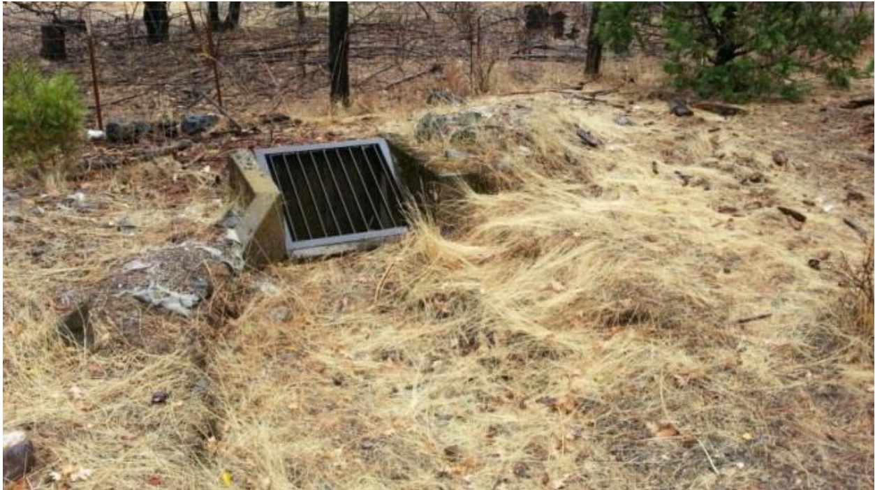
Figure 4-131 American Valley Localized Flooding – Small drain for Mill Creek can be Bypassed During Larger Storms Causing Water to Flow Down Adjacent Gravel Road.
