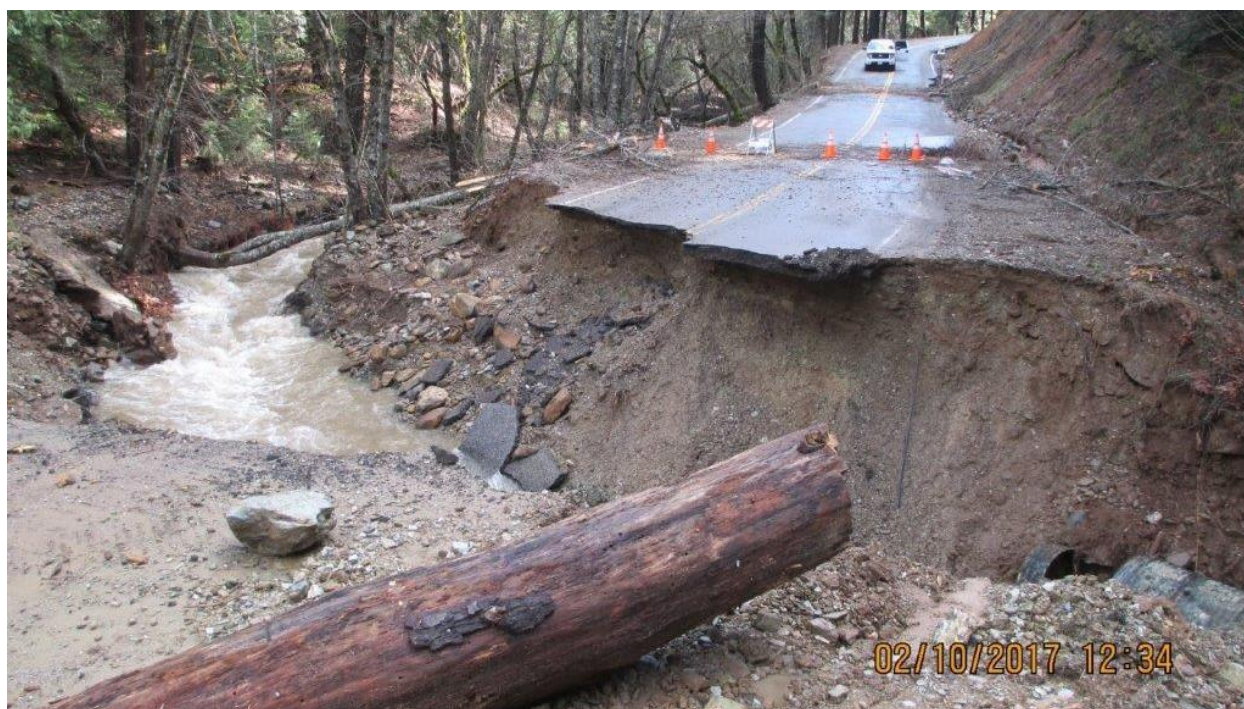
Figure 4-106 Plumas County – LaPorte Road Washout
