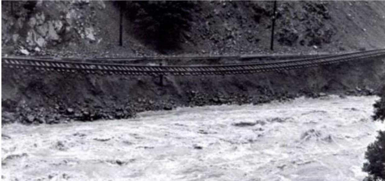
Figure 4-92 1986 Railroad Bed Flood Damages
