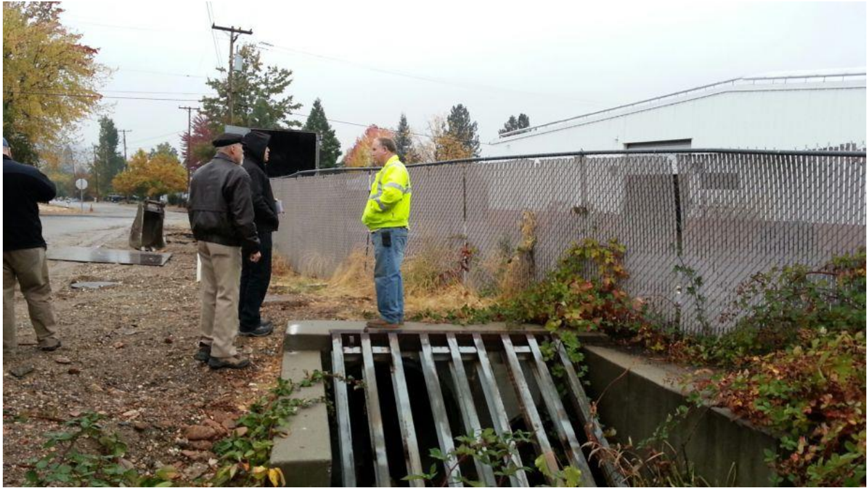
Figure 4-123 American Valley Localized Flooding – Storm Grate behind Les Schwab Becomes Clogged with Debris Causing Flooding
