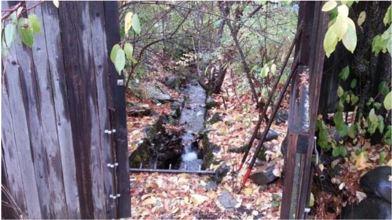
Figure 4-126 American Valley Localized Flooding – Hentschel’s Storm Grate, Small Grate for Localized Drainage Clogs with Debris and Causing Flooding over Roadway.
