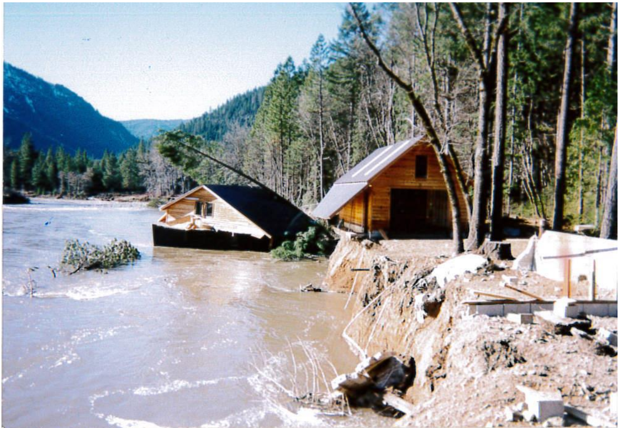
Figure 4-95 Erosion from Floodwaters Cause Home to fall into Indian Creek
