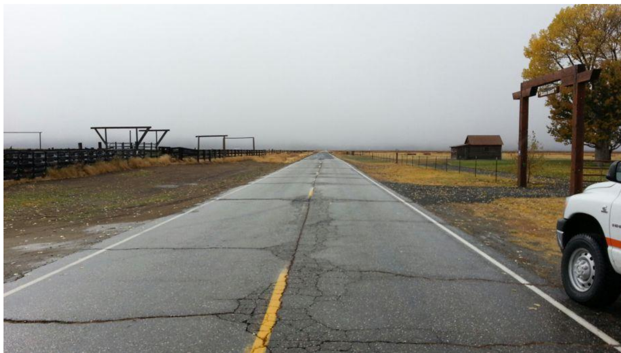
Figure 4-117 Harriet Lane – Pavement Deterioration from Localized Flooding
