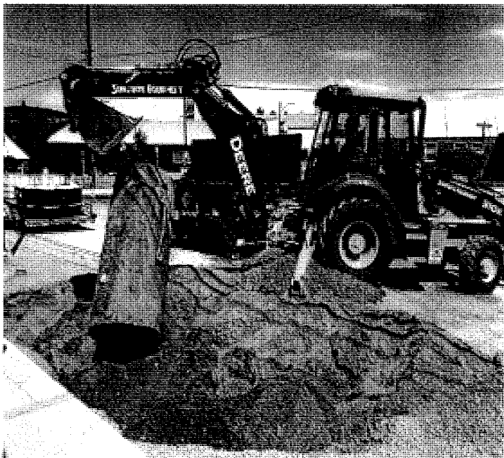
Underground Tank Removal, Pacific Street Portola
