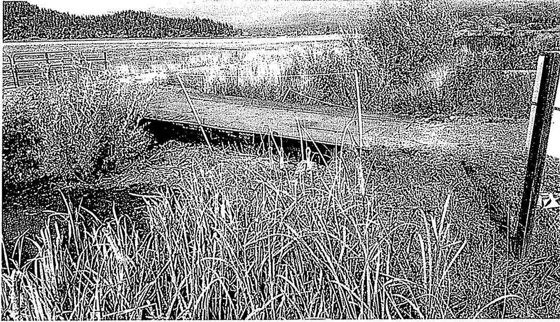
Crossing #1 (Debris stacked up against instream impoundments)
