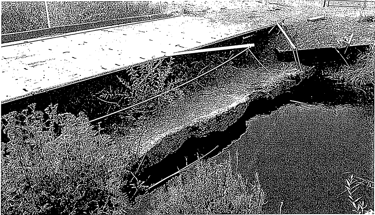
Crossing #1 (Two culverts located underneath concrete low-water crossing with flat car on top)
