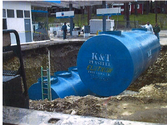
Underground Tank Installation at Graeagle Chevron
