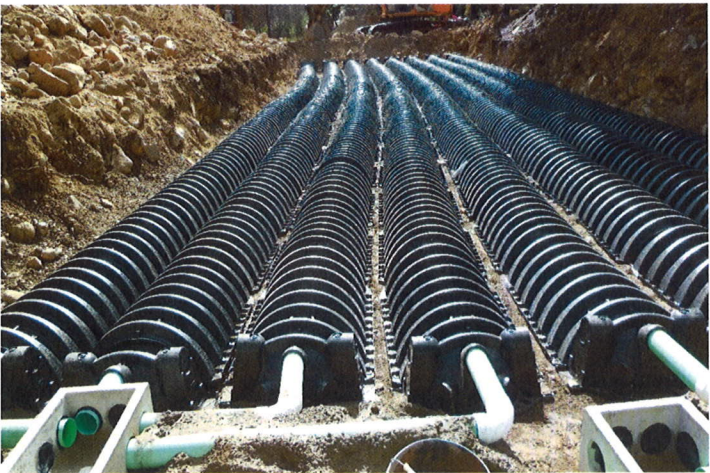
Gravel-less leachfield installation at North Fork Campground near Caribou
