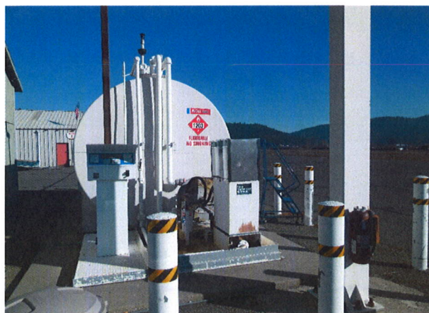
Above Ground Storage Tank at Gansner Airport
