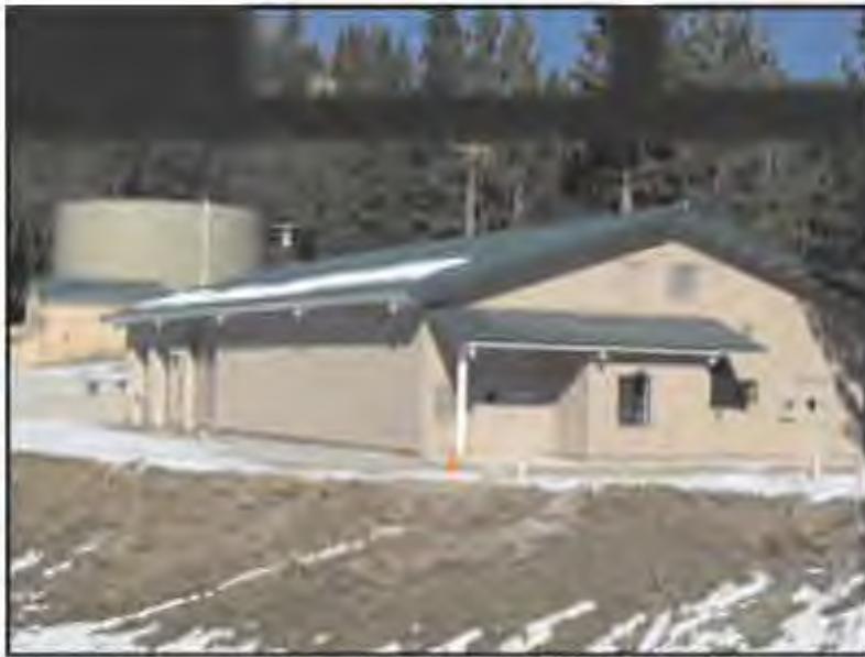
The Plant covers an area of approximately 10 acres and has a site elevation of 5,640 feet above mean sea level. The facilities include a water storage tank, a carbon filtration unit, a storage building, a filter building, two pressure filters, and two wastewater recovery ponds.
